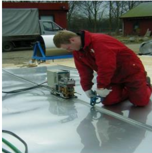
Figure 4. Induction welding of a stainless steel liner [5]
