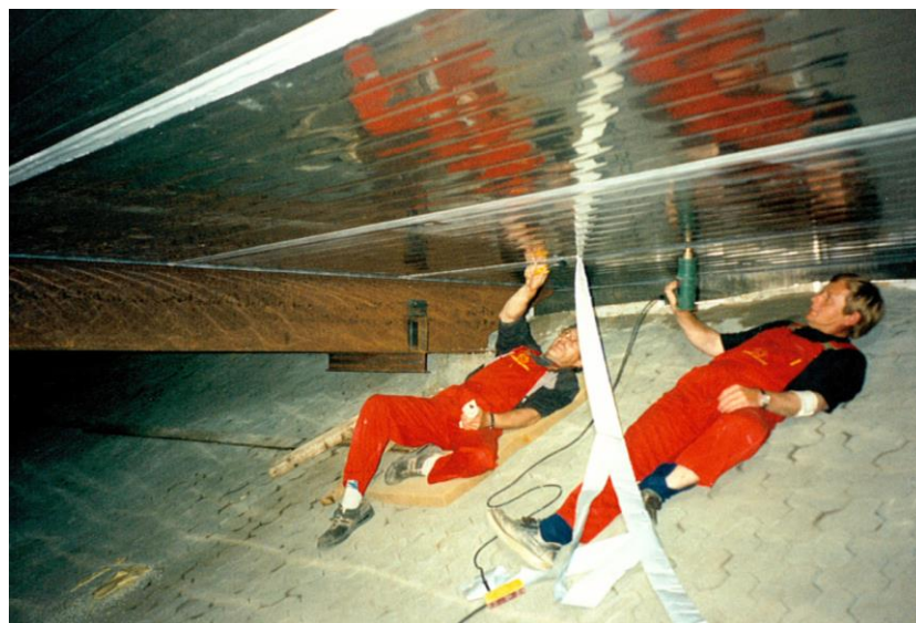
Figure 19 Sealing of joints on the water side [7].
